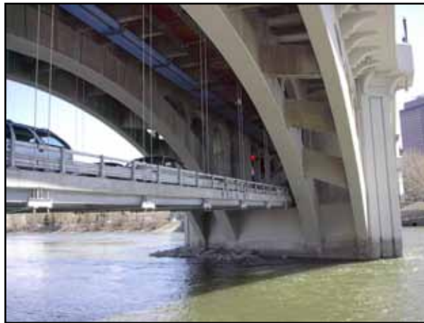
Figure 12.5: Lower Deck of Centre Street Bridge, Calgary, Alberta.
