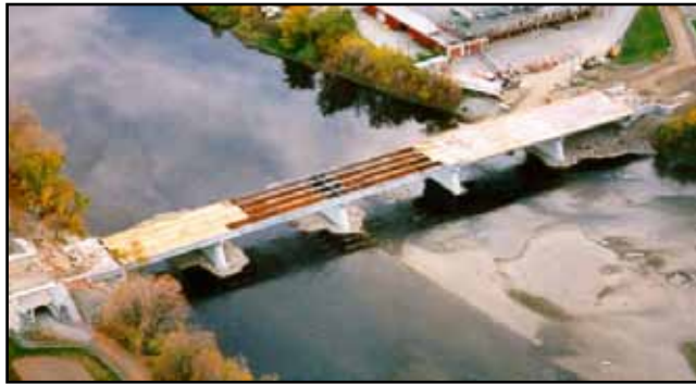
Figure 12.3: Aerial view of Joffre Bridge during construction.
